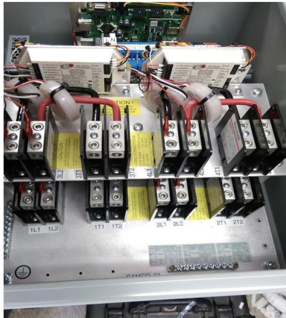
Relay-Meter Modules (RMM), by number "TB"=Terminal Block
